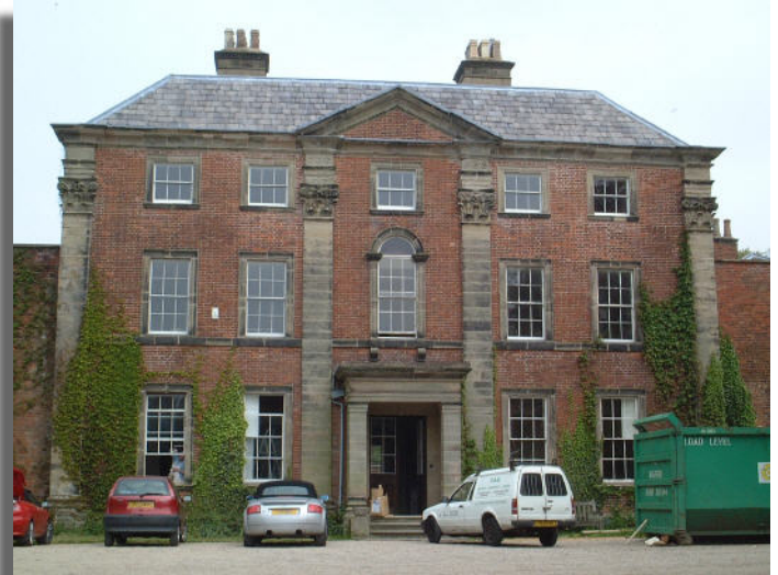
The facade before surveying
